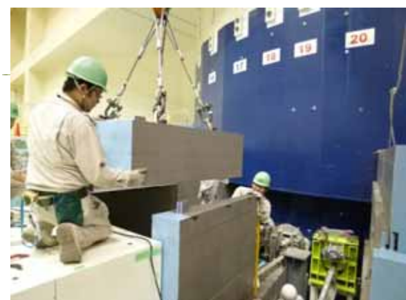
Reassembling of the shield device is in progress in the MLF. Fortunately the counter hall was not required for repairing.
