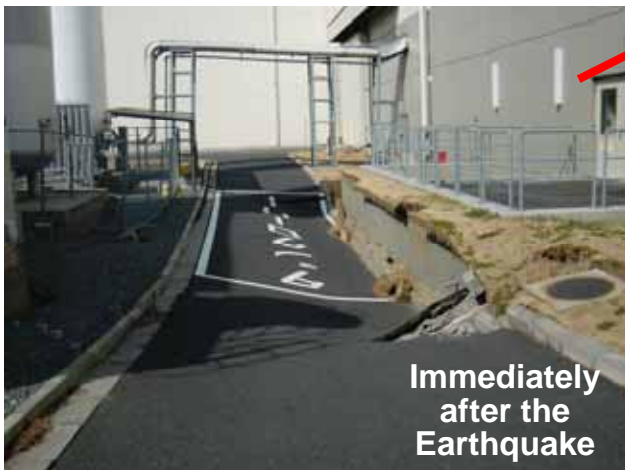
Immediately after the Earthquake Road at the west side of the MLF building felled in ~1.5 m
