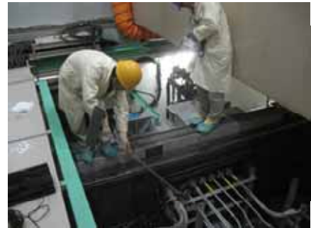
Measuring radiation level with opening a cover of the station.
