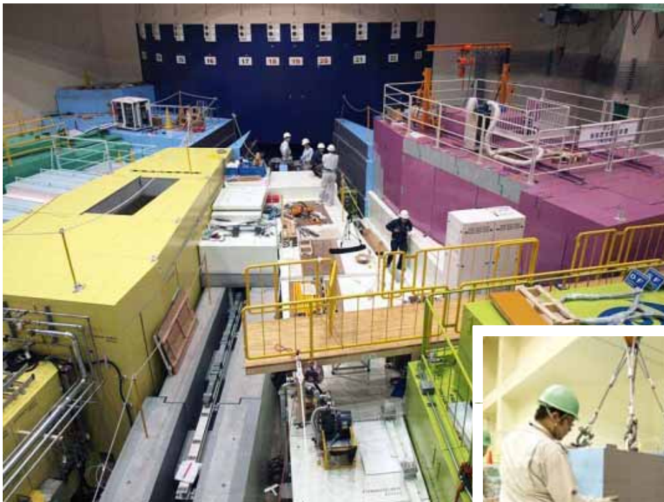
Reassembling of the shield device is in progress in the MLF. Fortunately the counter hall was not required for repairing.
