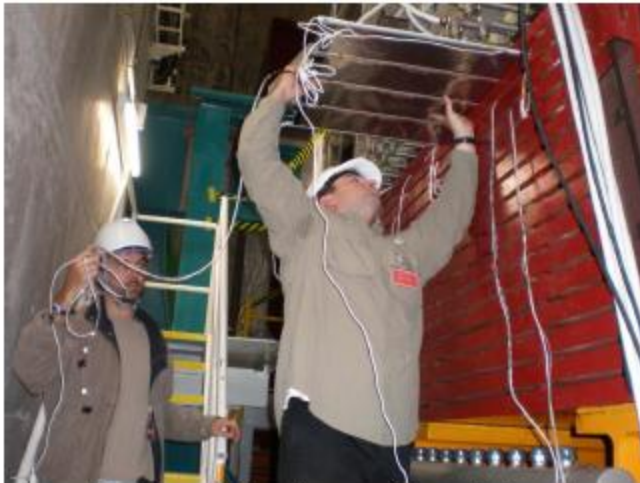
Installation of horizontal modules
